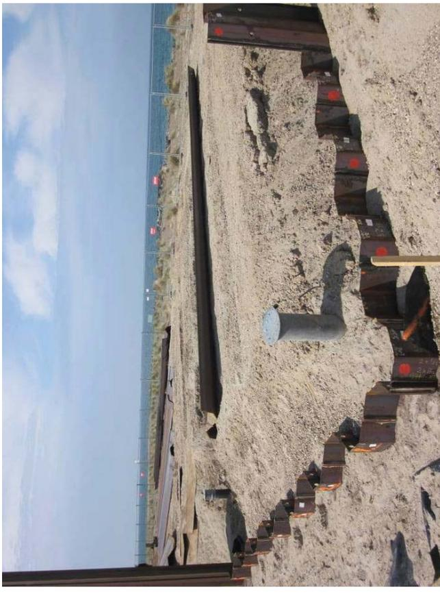
The main process in the experiments was to drain the test cells for natural groundwater and replace it with an alkaline NaOH solution (caustic soda), with pH 13. Over a few months the contaminants are degraded to less toxic water soluble compounds, which can be pumped up. This process was repeated twice. During the experiments it was closely monitored how much of the contaminants was degraded and how much of the contamination was removed.
